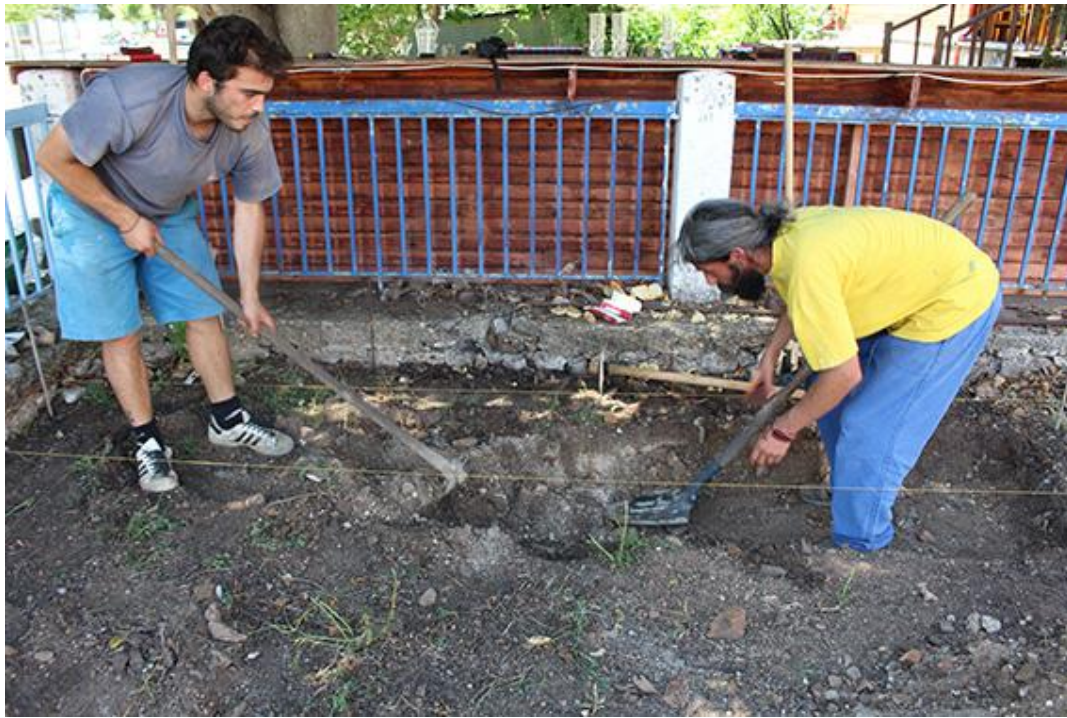
Digging for the foundations of the ceramic kiln, Prespes, 2016
